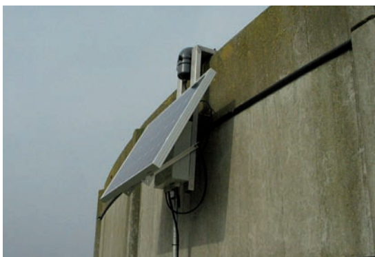
Photovoltaic driven alarm on a slurry tank.
