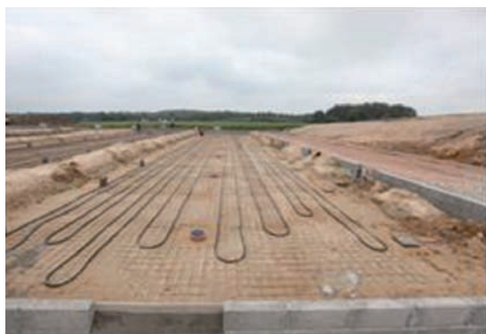
Tubes for slurry cooling laid out for being moulded into the slurry channel floors in a pig house to be built.
