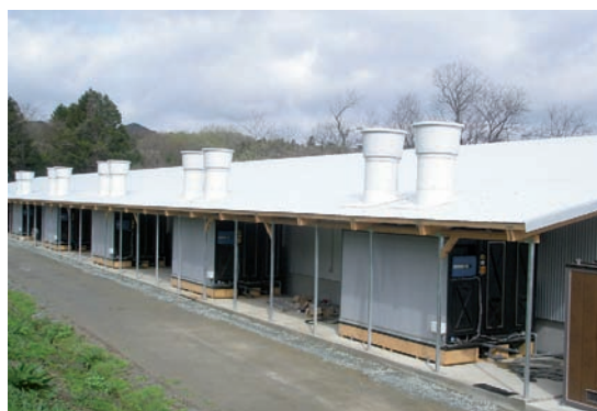
Biological air cleaning system being installed as part of the ventilation system in a pig house.
