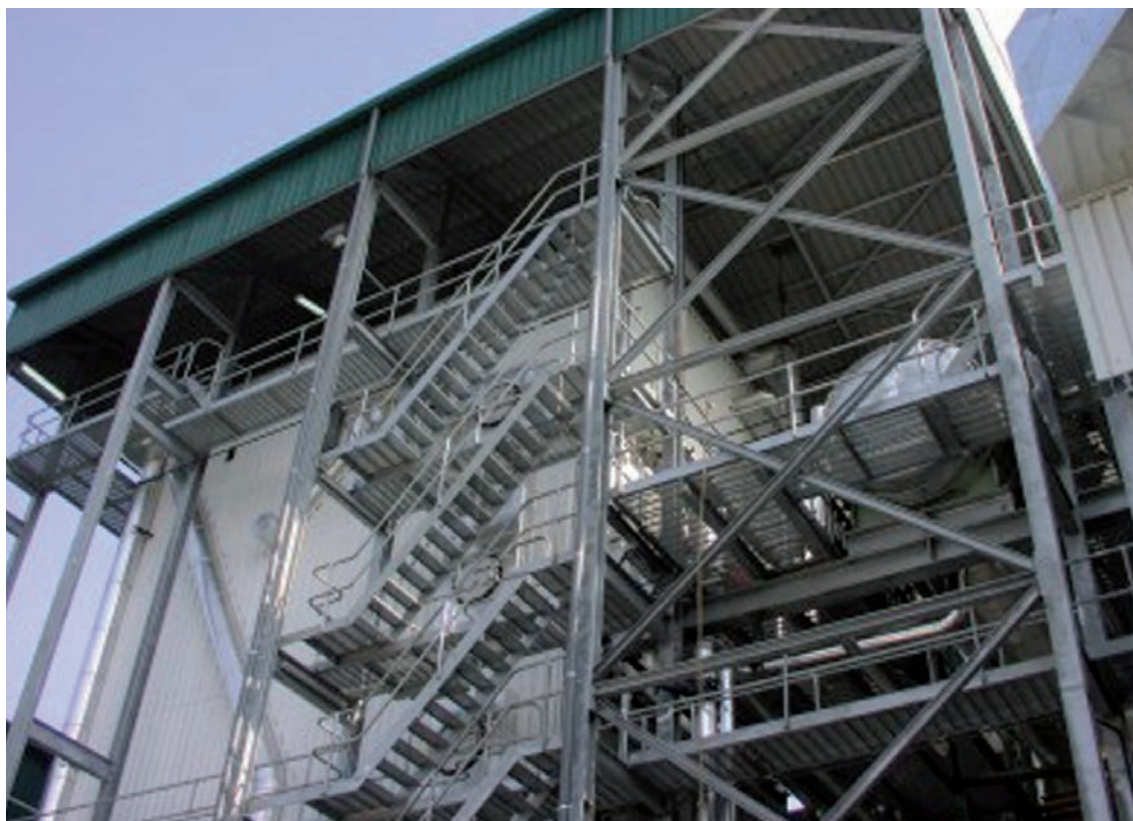
Industrial size boiler for combustion of chicken deep litter.
