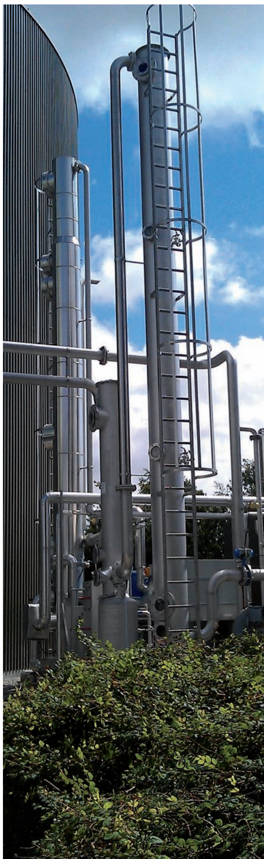
Upgrading of biogas to natural gas quality is mainly a question of separating methane from \text{CO}_2 and other unwanted gases. Here it is done in columns in a process based on amine absorption.
